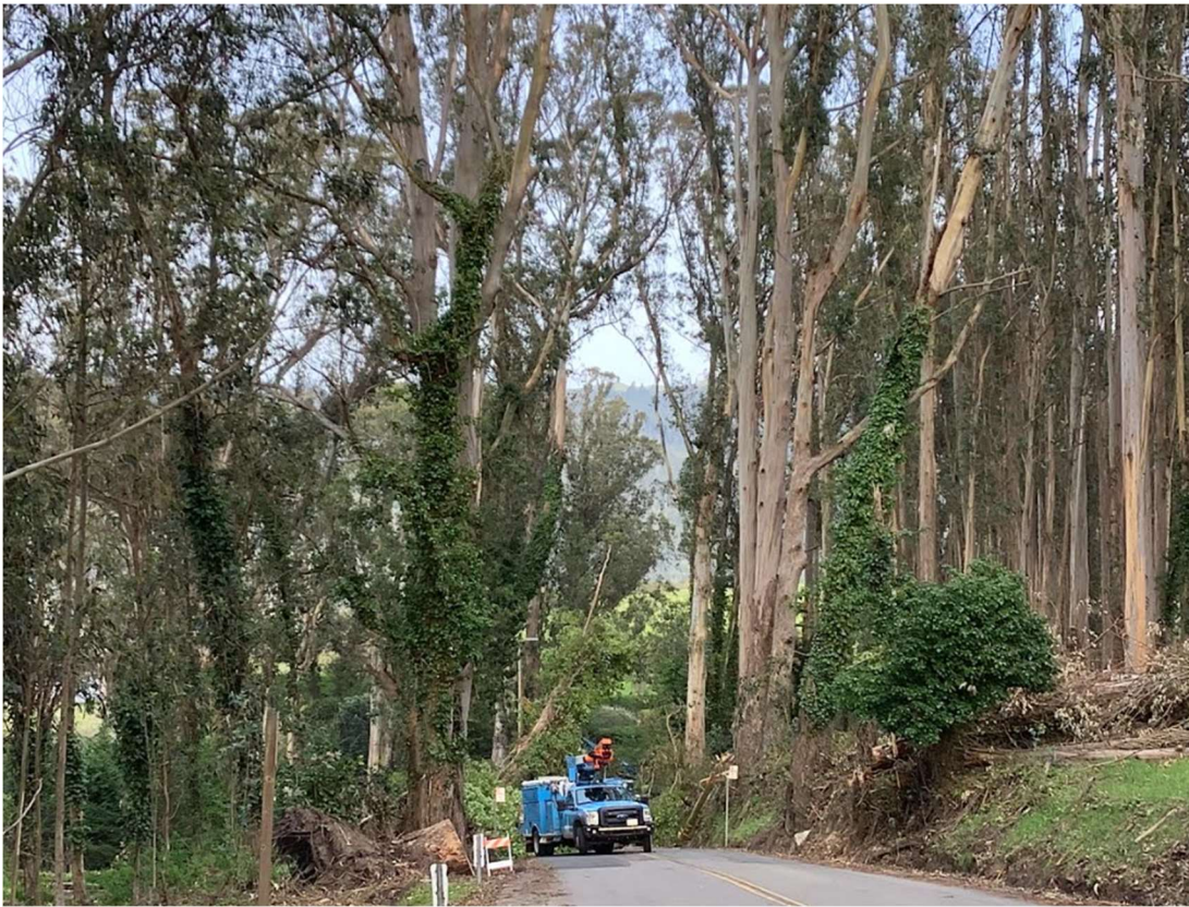
Figure 1 Zone 5 PG&E crews repair destruction caused by falling trees along Mesa Road
